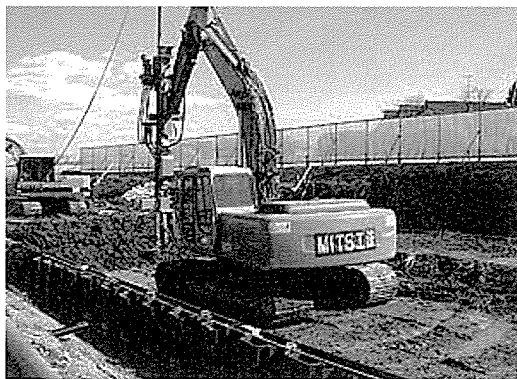
Fig.2 Construction of the MITS method
