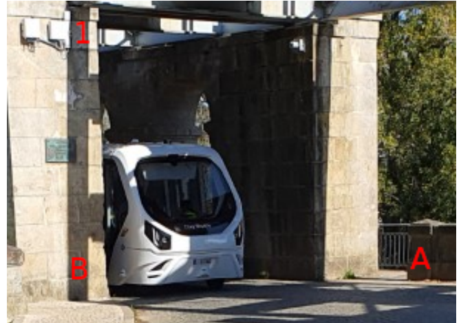
Fig. 2. Trial Location showing the shuttle about to leave the bridge
