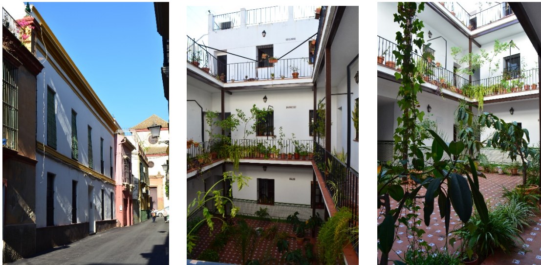
Fig. 3. Street view showing Calle Sagunto and the main entrance to the building (photo on the left) and images of the common inner patio, which provides access to the dwellings (two right-hand-side photos).
