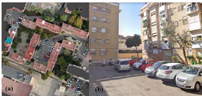
Fig. 5. (a) Aerial view of the social housing blocks. (b) Block type under study (Saeta Street 1) Source: Authors' own.
