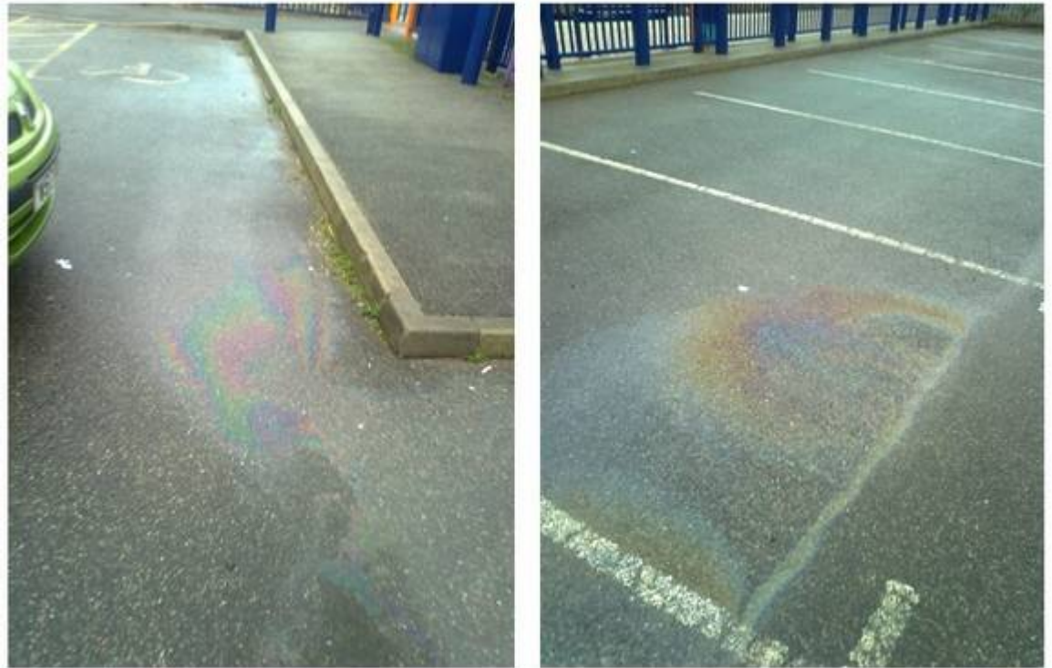
Figure 3: An example illustrating the fact that despite recent improvements in oil seal technology the loss of hydrocarbons onto car park surfaces can still be important (photographs taken by the candidate Jan. 2012, Whitwell Railway Station, Derbyshire).
