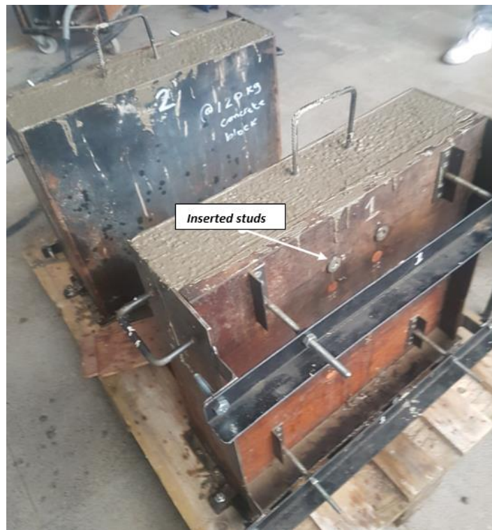
(a) Concrete infilled into Fabricated Mould
