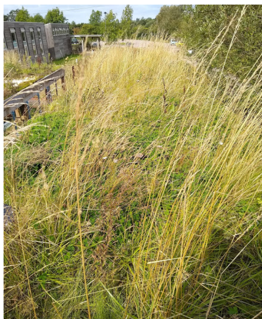
Figure 1. The surface of the blue green roofs from where runoff was collected.
