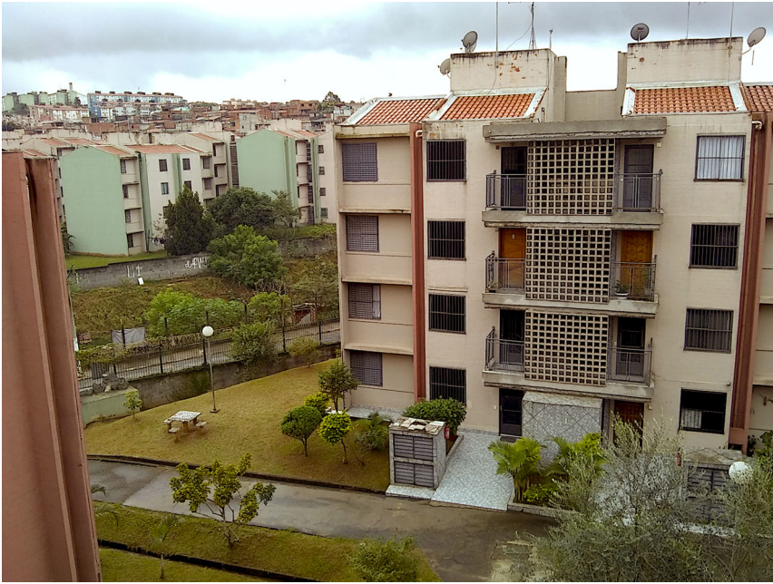
Figure 1 Mutirão housing in Fazenda da Juta. Photo credit: Matthew Richmond, May 2019.
