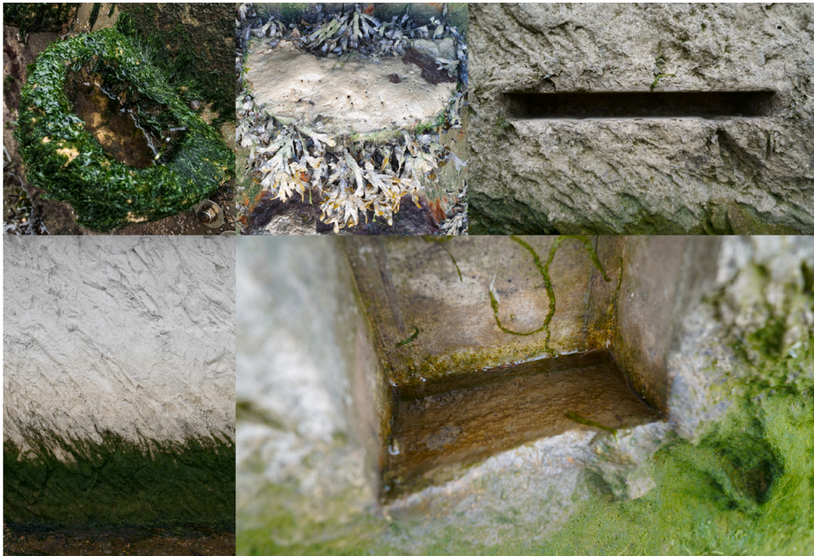
Fig. 2. Examples of coastal eco-engineering. Top left, clockwise: An artificial rockpool containing water (Marineff Project); a Vertipool containing mud (Bone et al., 2022); a ‘letter box’ crevice in a concrete seawall; a cubic void containing water in a concrete seawall; a concrete seawall with a ‘rockface’ textured surface created with a formliner. Images by Jessica R. Bone.
