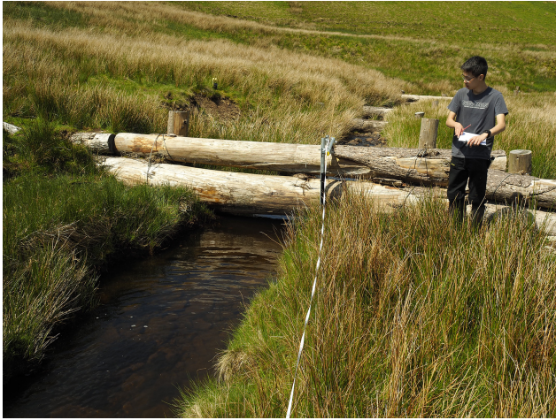
Figure 1. Jam 16 of 77 installed at Tebay Gill, Cumbria.
