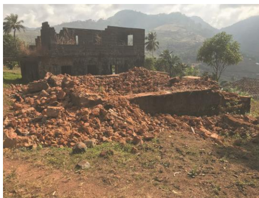
Figure 3.4b: The stone house pictured in 3.4a after demolition (circa January 2021). (Source: Photograph by the Author)
