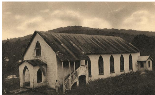
Figure 1.8b: St. Charles Parish at Regent Village before renovation. (Source: Special Collections, Yale Divinity School Library)
