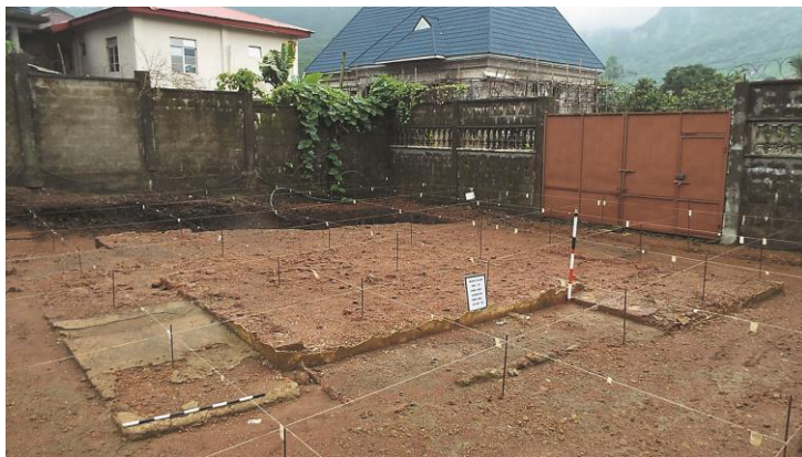
Figure 4.9a: The extent of the main house structure. (Source: Photograph by the Author)
