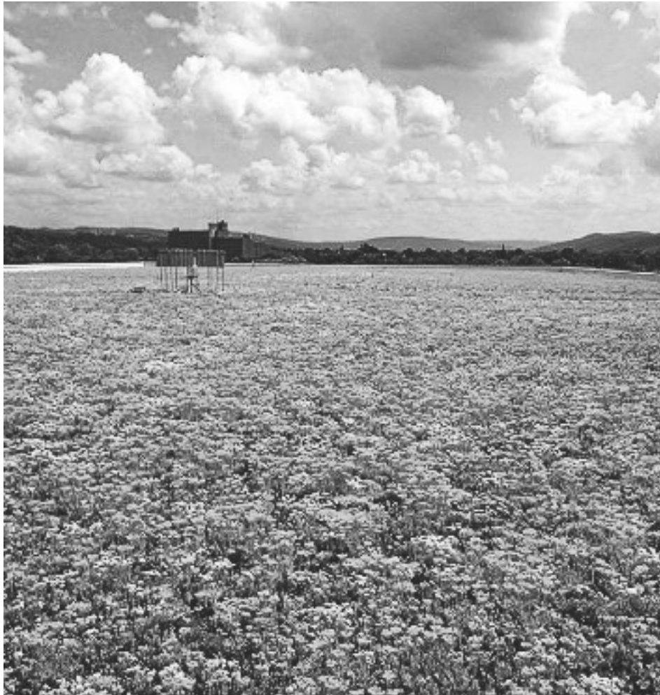
Figure 2.1 Looking south on the OnCenter green roof during the Summer 2013. The Belfort AEPG 1000 precipitation gauge and altershield are seen in the left side of the image while additional instrumentation on tripods is barely visible at the other end of the large roof.
