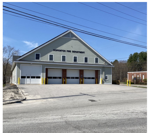
Hopkinton Fire Station
