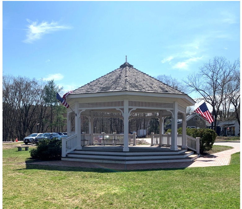
Gazebo at Riverway Park along the Contoocook River
