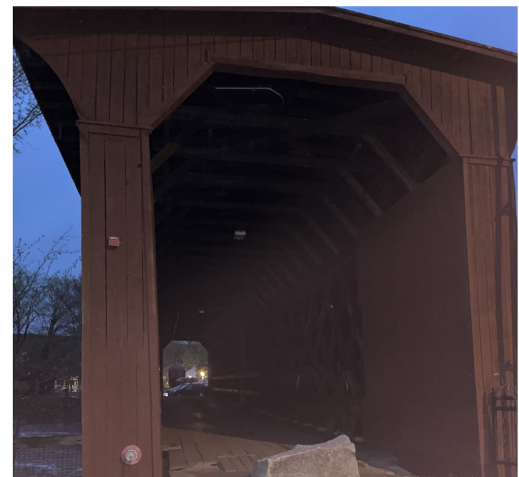
Unlit railroad bridge
