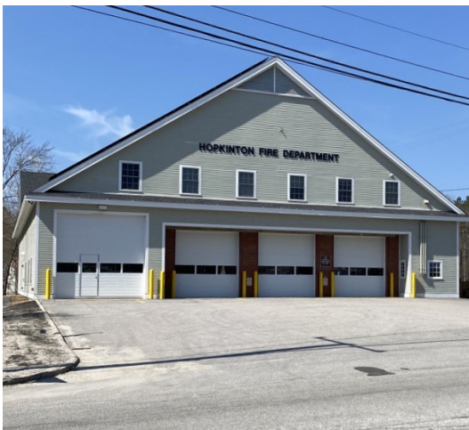
Hopkinton Fire Station
