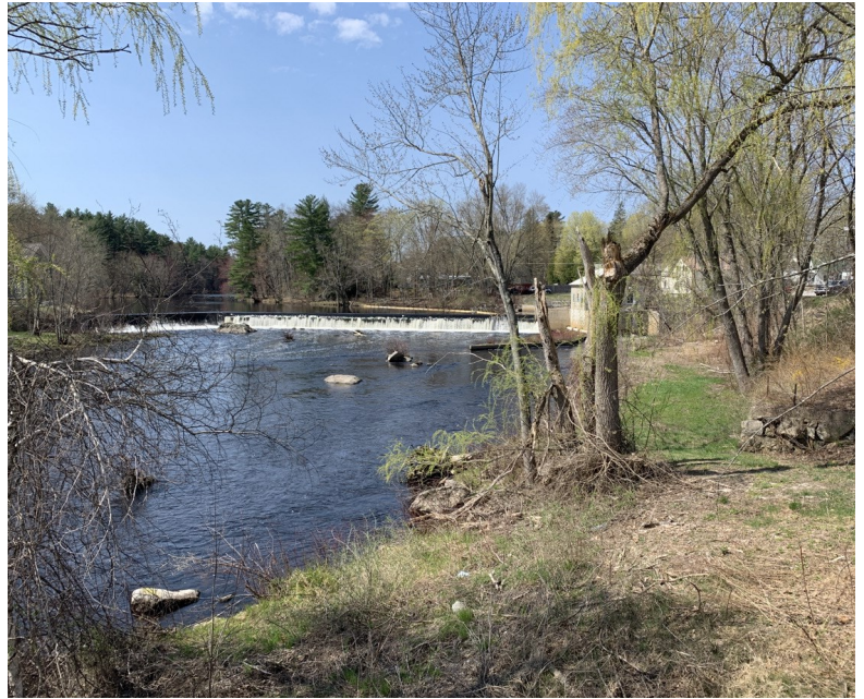
Tree trimming needed to enhance view of Contoocook River and dam
