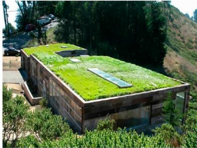
Figure 2: Extensive green roof [25].
