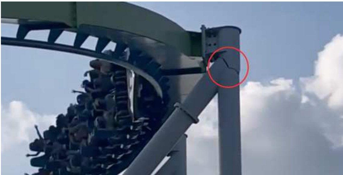
Figure 1.1: Example of Fatigue Failure on roller coaster. North Carolina, 30/06/23, Corriere.it
