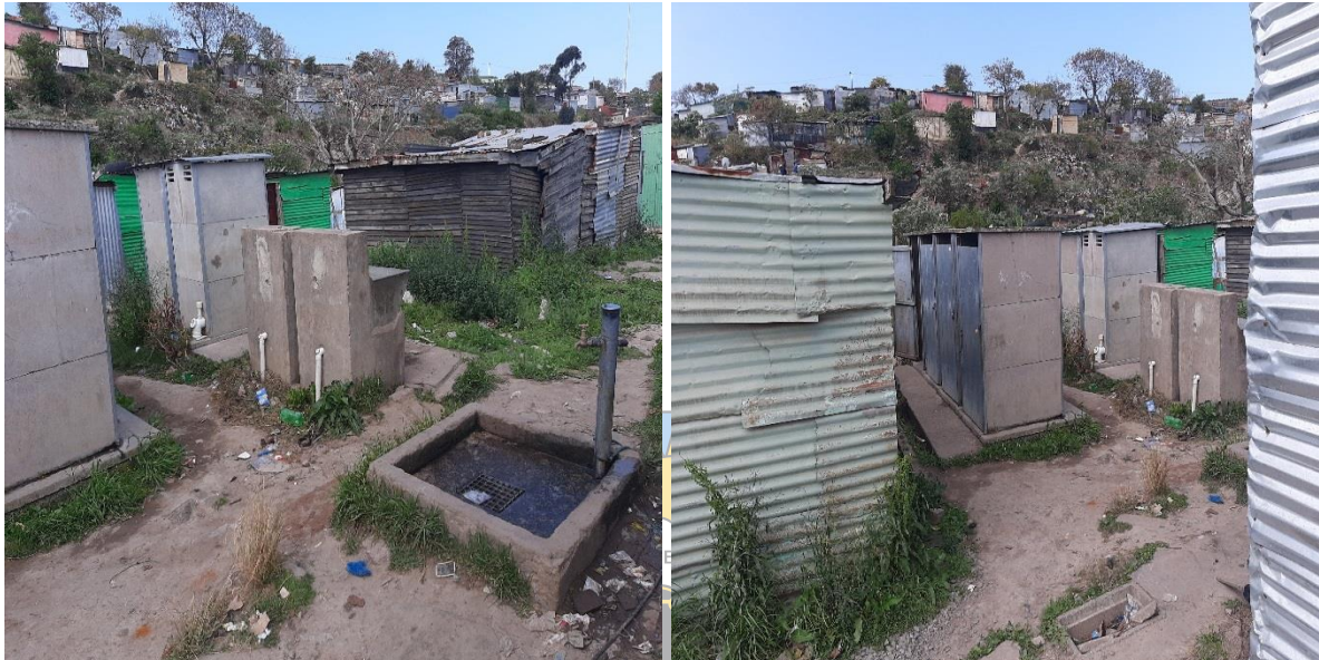
Figure 26a & b: Showing examples of water standpipes and communal ablution facilities in Ward 8, Duncan Village. Source: (Author, November 2021)
