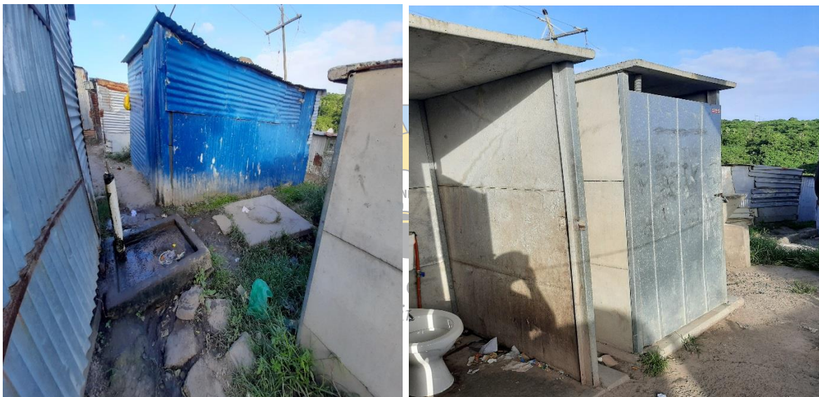
Figure 24a & b: Showing examples of communal standpipes and communal ablution facilities both in Ward 6, Duncan Village. Source: (Author, November 2021)
