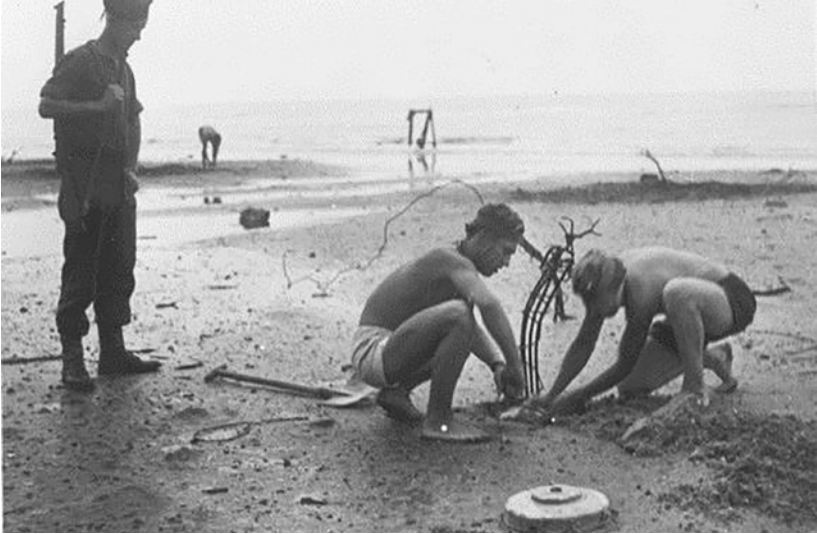
Tellermine-42s being removed from beach obstacles using clearance drills acceptable at the time. Tellermine coated in tar were found to be resilient to seawater for up to six months. Image: NIOD Institute
