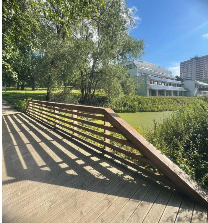
Figure 21. Focus area 1 picture (the bridge number 2) (Used with permission of Shaik Muhammed Zubair Basheer Ahamed, 2023)
