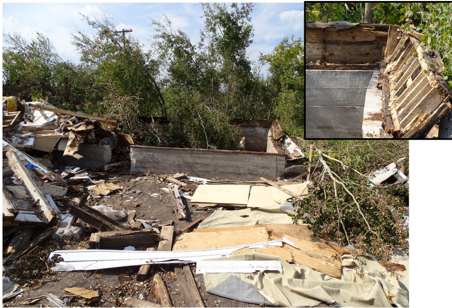
Fig. 4. Damage to abandoned residential structure at Site 2, assessed as DOD9 of FR12. Inset shows closer view of remaining knee wall.
