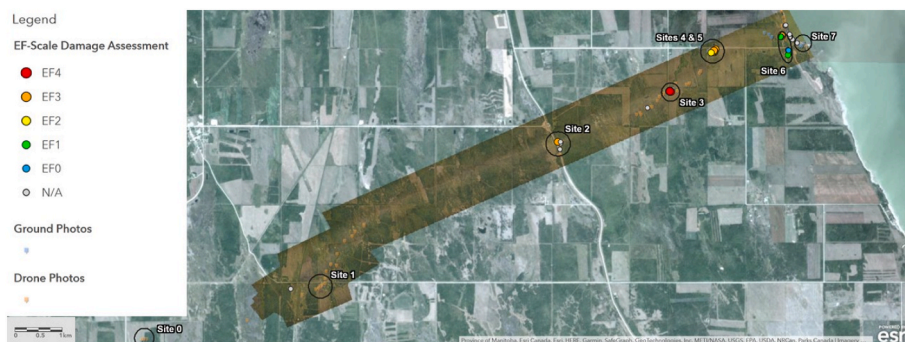
Fig. 1. Overview of Alonsa tornado path as viewed with satellite imagery, with ground survey sites with EF-Scale assessments of structural damage labelled.
