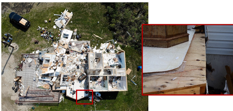
Fig. 6. Drone image of DOD8 damage at Site 5. Inset shows edge of floor structure; exposed plywood indicates location where walls used to sit.
