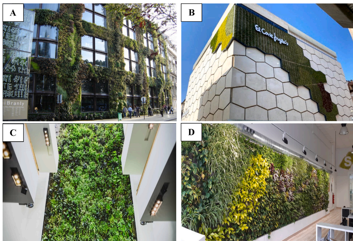
Fig. 5. Examples of botanical filters. A. Musée du Quai Branly – Paris, France. B. Outdoor vertical garden in Corte Inglés - Valladolid, Spain. C. Biofilter of the University of Guelph's central atrium – Humber, Toronto. D. Singular Green Company – Alicante, Spain.
