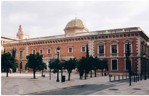
Fig. 11. Cultural Centre 'La Nau' where the LoRa monitoring system was installed.
