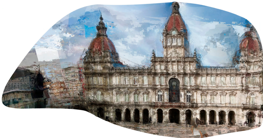
Figure 6: Orthoimage of the mesh on the collective vision of the facade of the town hall square in A Coruña using photogrammetry techniques in the Autodesk Recap Photo software, the authors, 2022.
