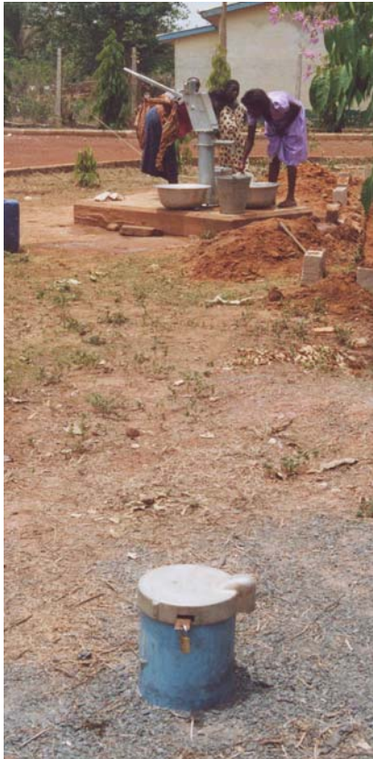
Capped exploration Bh No.2 at Tease and pumping APDO Bh.
