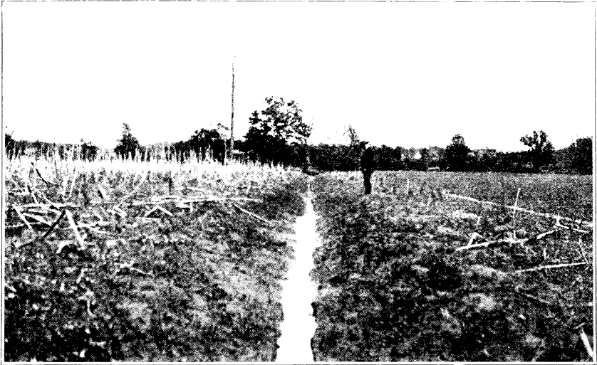
Fig. 5.—Ditch blasted with dynamite cartridges 1\frac{1}{8} by 8 inches in size. Cape Girardeau county.
