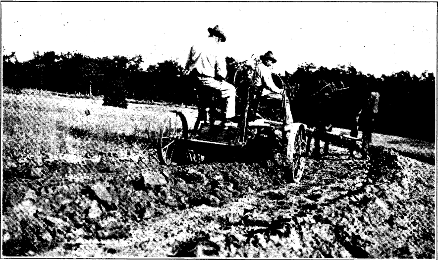
Fig. 7.—Last round with the grader in building a soil saving terrace in Perry county.
