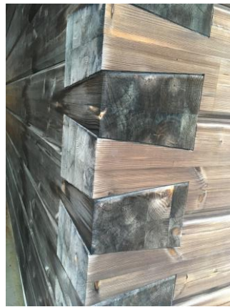
Figure 3. Dovetail connection detail in a wall.
