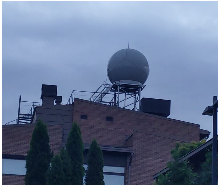
Figure 3.1. WRS400 on the roof of Vaisala headquarters in Vantaa.
