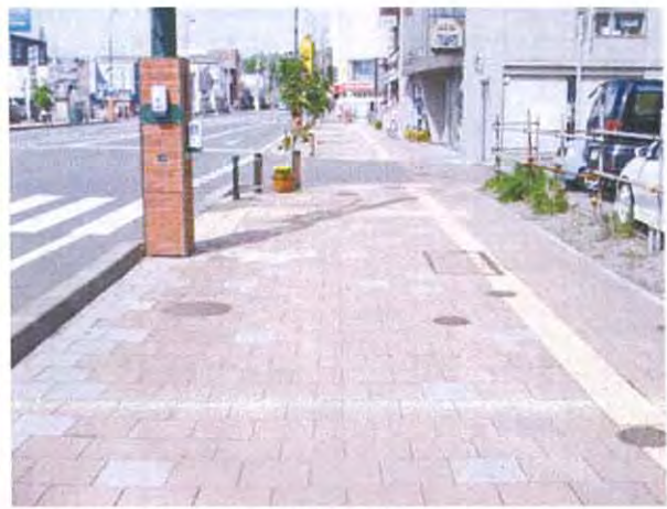
Photo 4. After Barrier Free Improvement
