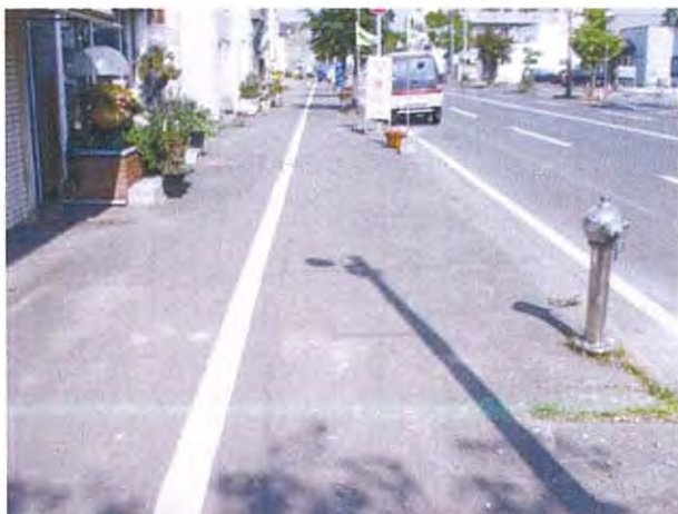
Photo 3. Before Barrier Free Improvement
