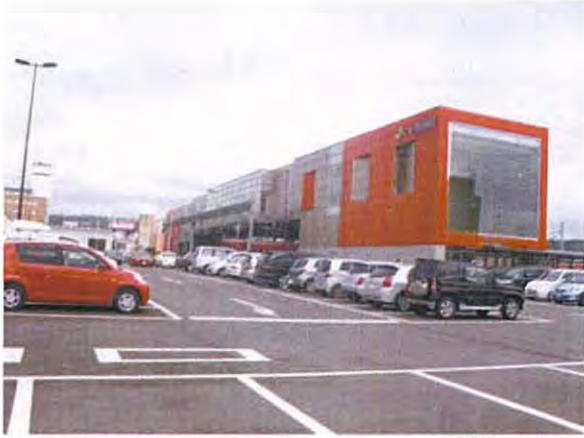
Photo 1. Design of the New Passage of Higashi-muroran Station
