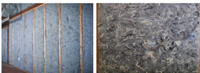
Figure 2. Wall claddings made of recycled denim (left) and cotton (right) [8].
