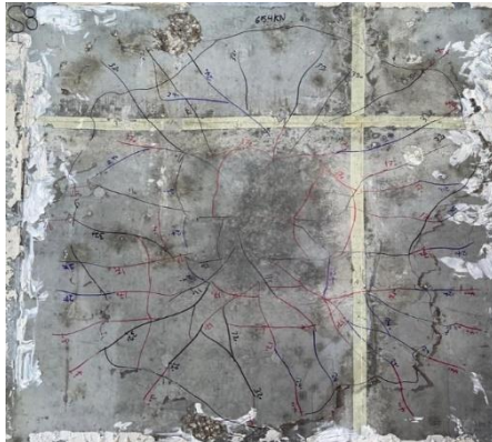
(h) Crack patterns of S8
