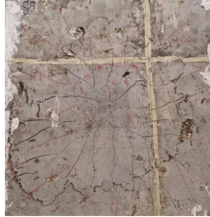
(e) Crack patterns of S5
