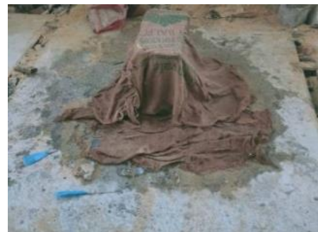
(c) Casting and curing of SHCC hidden capitals and the column
