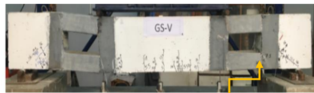
(a) Debonding of GFRP
