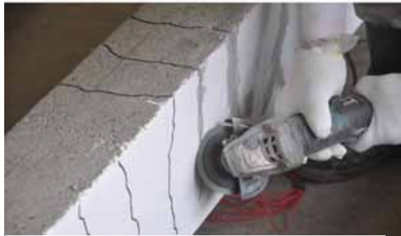
(a) Preparing the cracks surfaces
