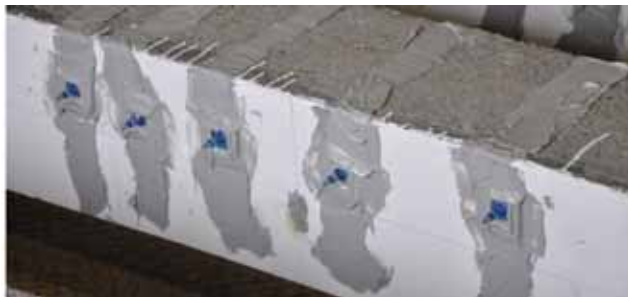
(c) Coating the cracks surfaces with putty
