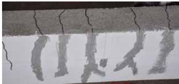
(a) After preparing the cracks surfaces
