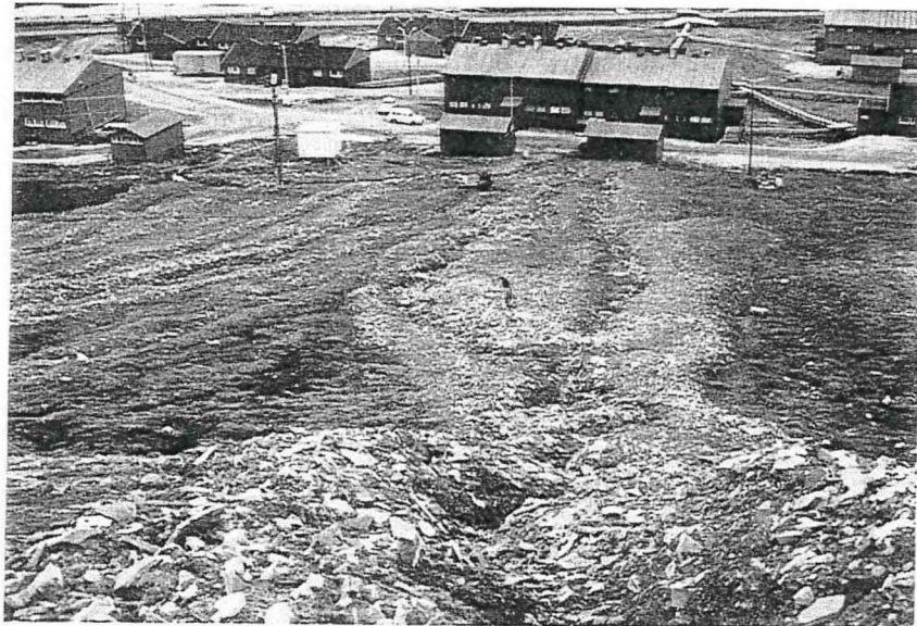
Figure 8: Houses along road 226 are located on debris flow deposits.
