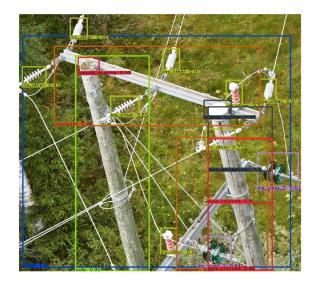
Figure 3.3: Detection of different components of a utility pole Image credit: [10]
