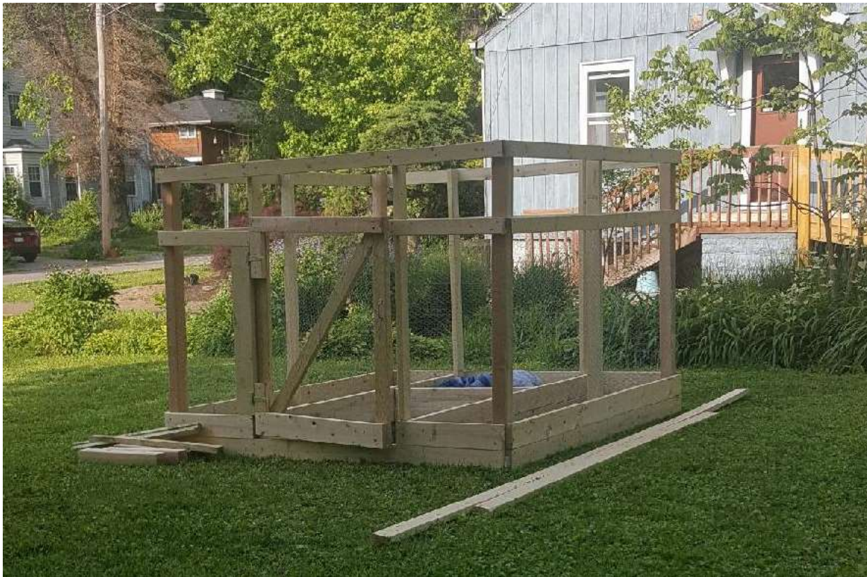
Figure 10. Francine and Al's enclosed beds during construction. Photo by Francine.
