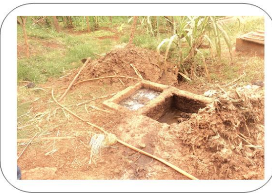
Fig. 2. Biogas plant at Viti village indicates poor management that lead to low gas production and destruction of the plant system.
