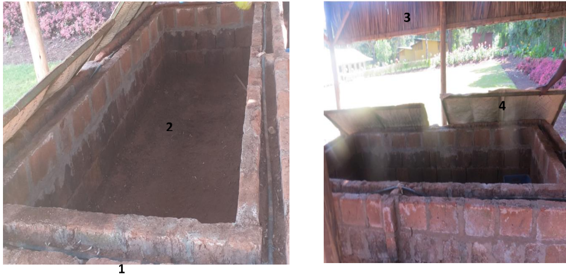
Plate 3: Traditional vegetable cooling chamber (a) or zero energy cooling chamber (b): (1) water circulating chamber with pipes used to distribute water; (2) cooling chamber, where vegetables are preserved; (3) grass thatched to protect heat and direct sunlight; (4) the rid or cover, made with bamboo leaves
