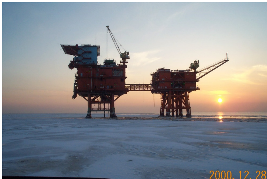
Figure 5 JZ20-2 oil platform in Liaodong Bay (photograph supplied by Ji Shunying).
