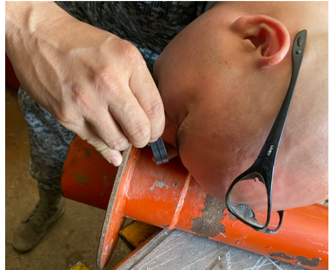
Figure 15 Visual inspection of the anchorage structure using a 10× magnification lens.
