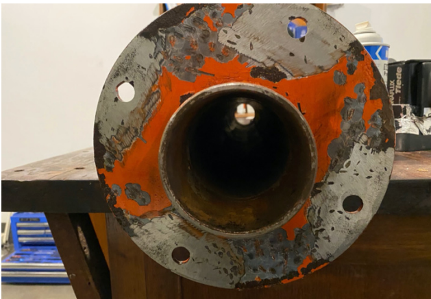
Figure 17 Support of the wind turbine tensor cable prepared for inspection.
