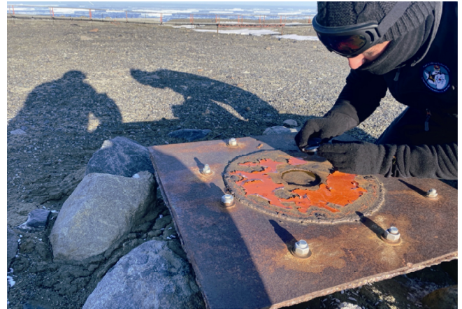
Figure 22 Visual inspection of the turbine base using a 10× magnification lens.
