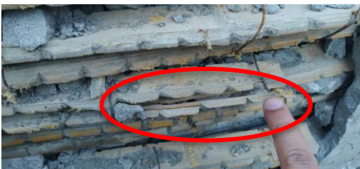
Figure 12: Splitting of tension bamboo.
