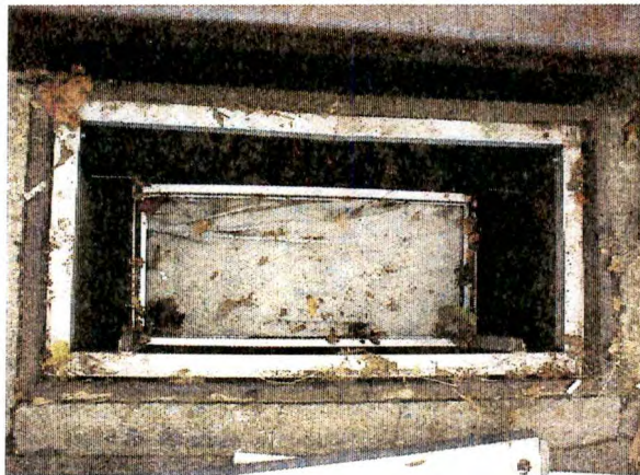
Figure 5-8. Philip Fulmer Way Inspection Photo
