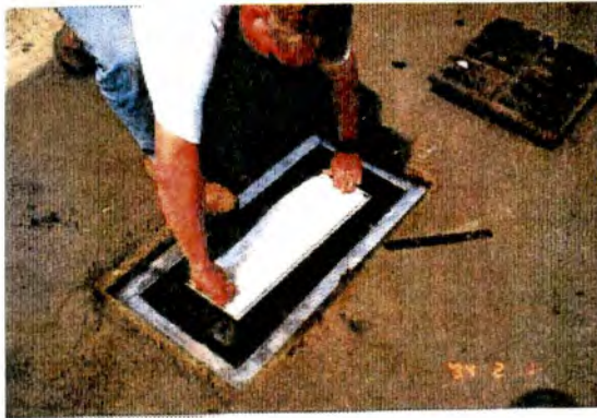
Installation of Filter Media
