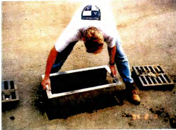
Placement of Stainless Steel Housing
