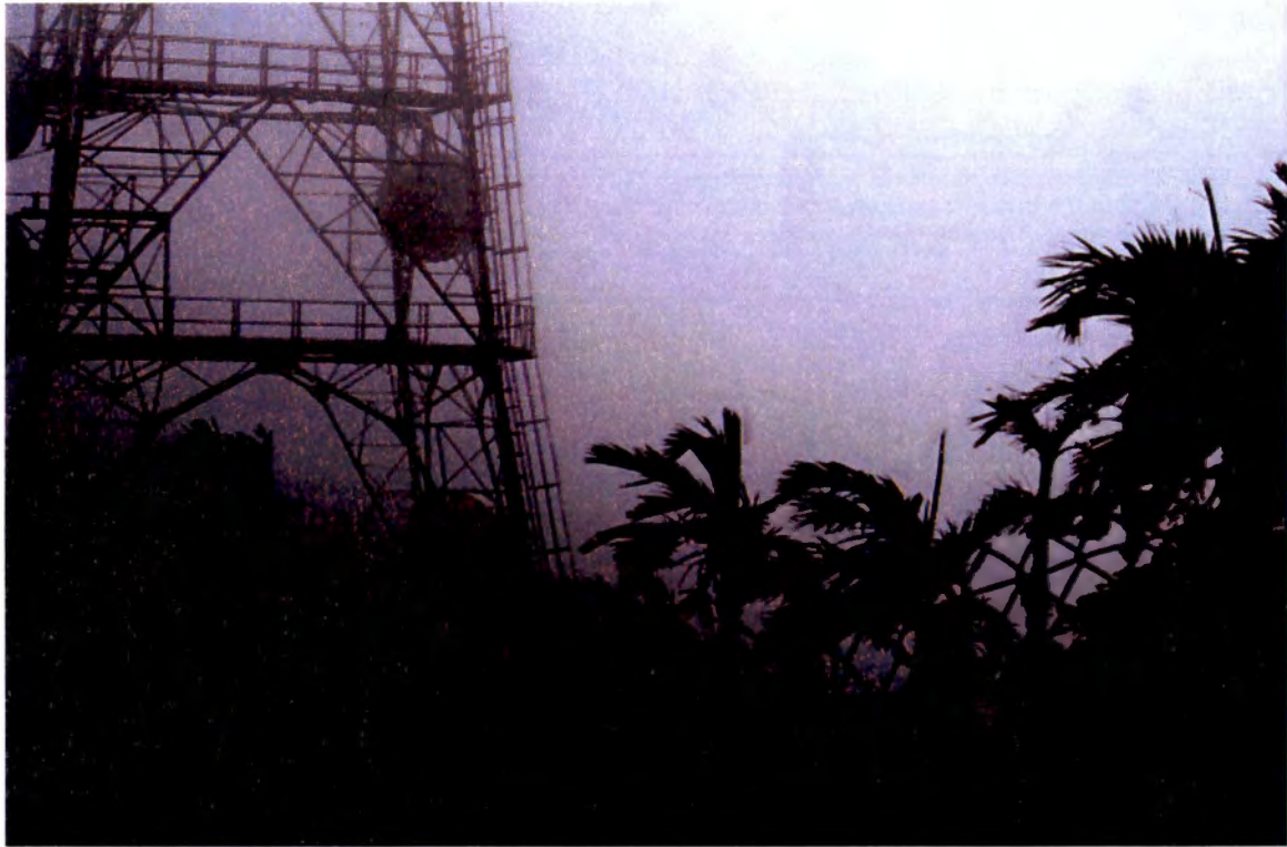
Figure 3-6. The Cable and Wireless tower sits enveloped in clouds on Chances Peak, Montserrat. Rising 65 m above cloud forest, the tower supports seven satellite dishes and provides telecommunication services to the island.
