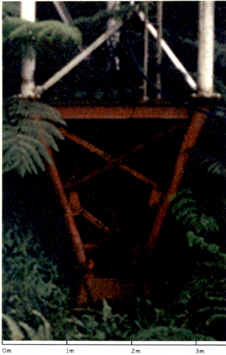
Figure 3-7. The base of the Antilles Television antenna on Chances Peak, Montserrat, measures one square meter. The massive antenna was originally used for intercepting television signals emanating from other islands in the Lesser Antilles. Today it is used for transmitting FM radio.
