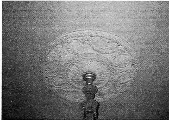
Figure 49. Ceiling medallion in main parlor of Cannon-Stickley Home
