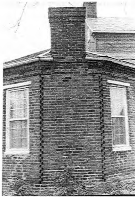
Figure 17. Back view of Cooke-Kefauver residence Madisonville, Tennessee.
