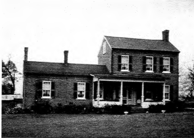
Figure 9. Coffin-Turner home prior to 1981 renovation.
