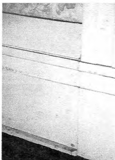
Figure 43. Baseboard molding Cannon-Stickley Home
