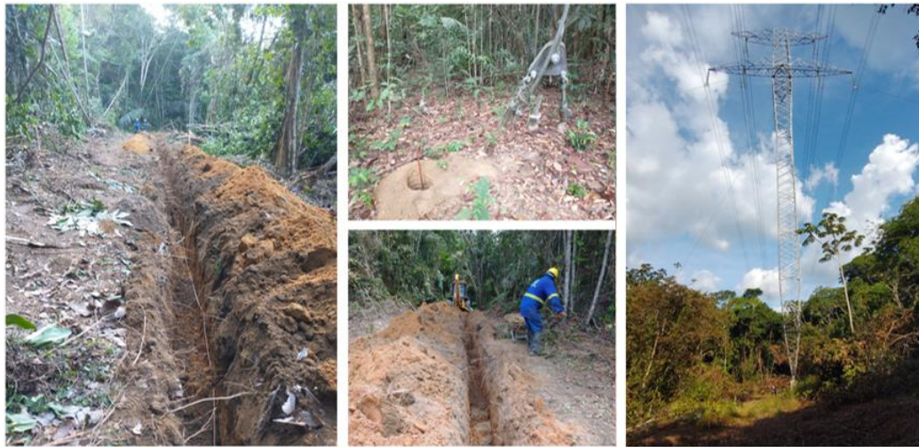
Picture 8. Execution of the activities on site.
