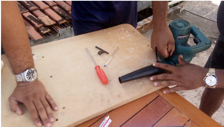
Figure 2 - Blower fixation on the MDF board.
