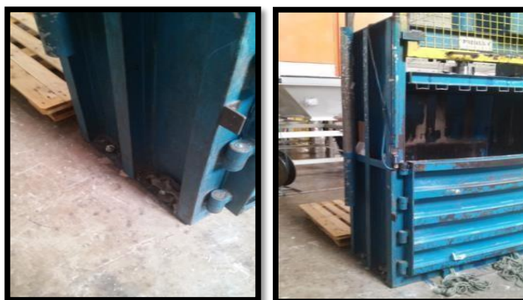
Figure 8 - Fixing the machinery.
