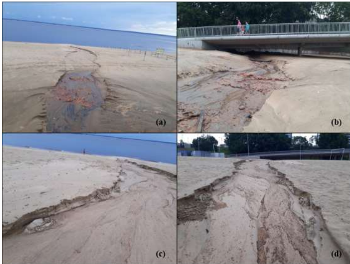
Figure 8: Features found on the landfill surface during low water periods, in 2018 - Features of sandy movement due to rain. Photos a and c) show the sediments towards the river, and photos b and d) show the sediments coming from the beach.
