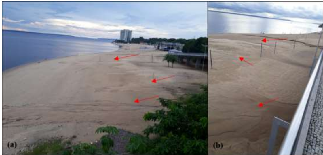
Figure 11: Features found on the landfill surface during low water periods, in 2019 - a) and b) Beach surface presenting, in general, the sandy mass movement features.
