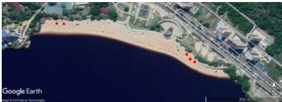
Figure 10: Places where the movements of sandy masses in figures 7, 8 and 9 occur, and water accumulation in figure 7a, caused by the presence of pipes and stairs that channel rainwater more intensely.
