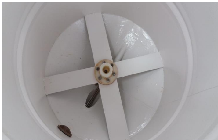
Figure 15. Internally painted reactor drum.
