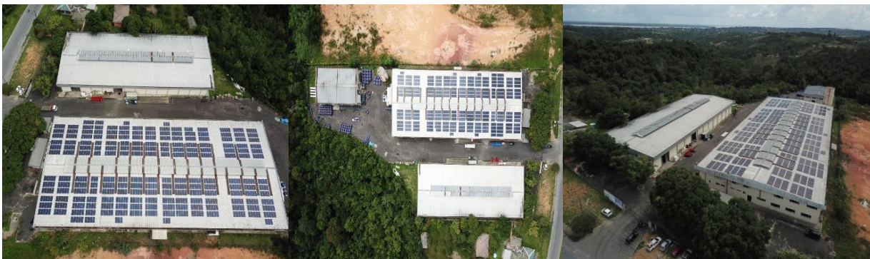
Figure 2. Factory with solar system installed.
