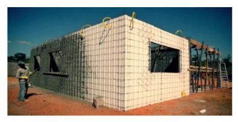
Figure 05: Application of microcement with equipment
