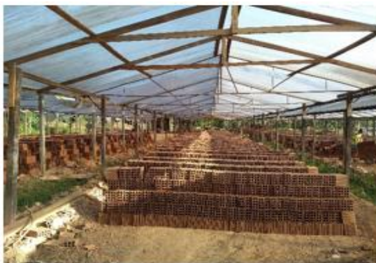
Figure 13: Internal drying area
